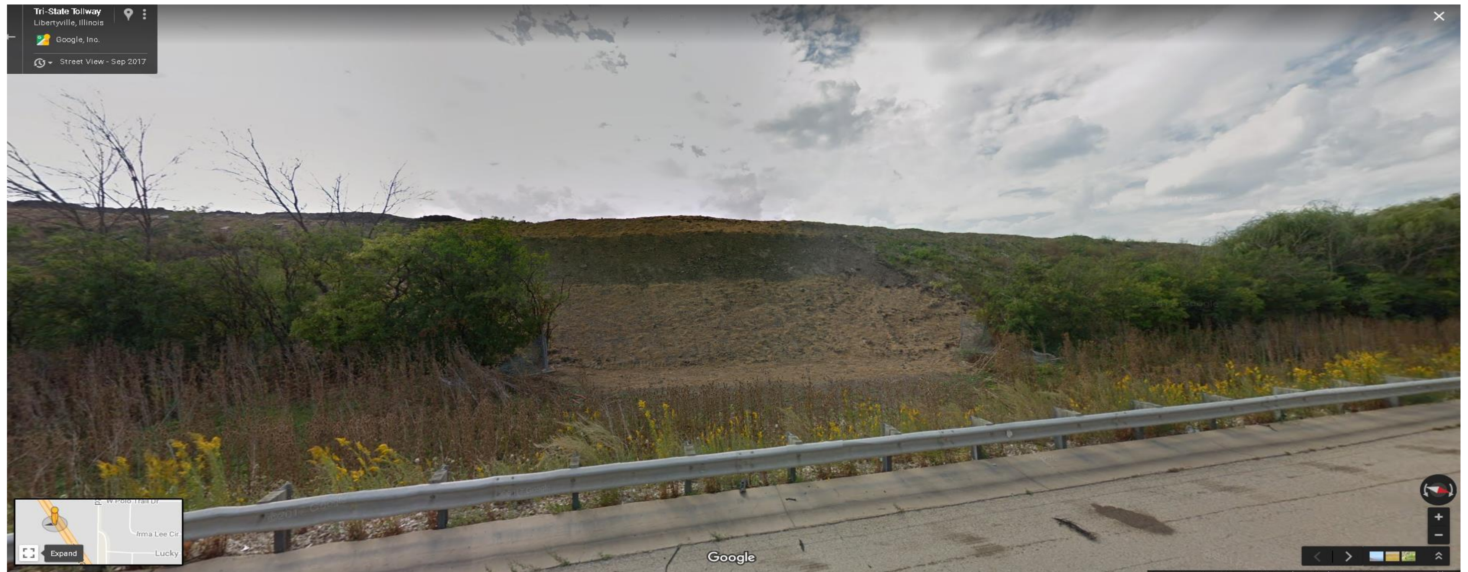
Figure 1: Google Street View of Berm Failure into I-94 ROW
