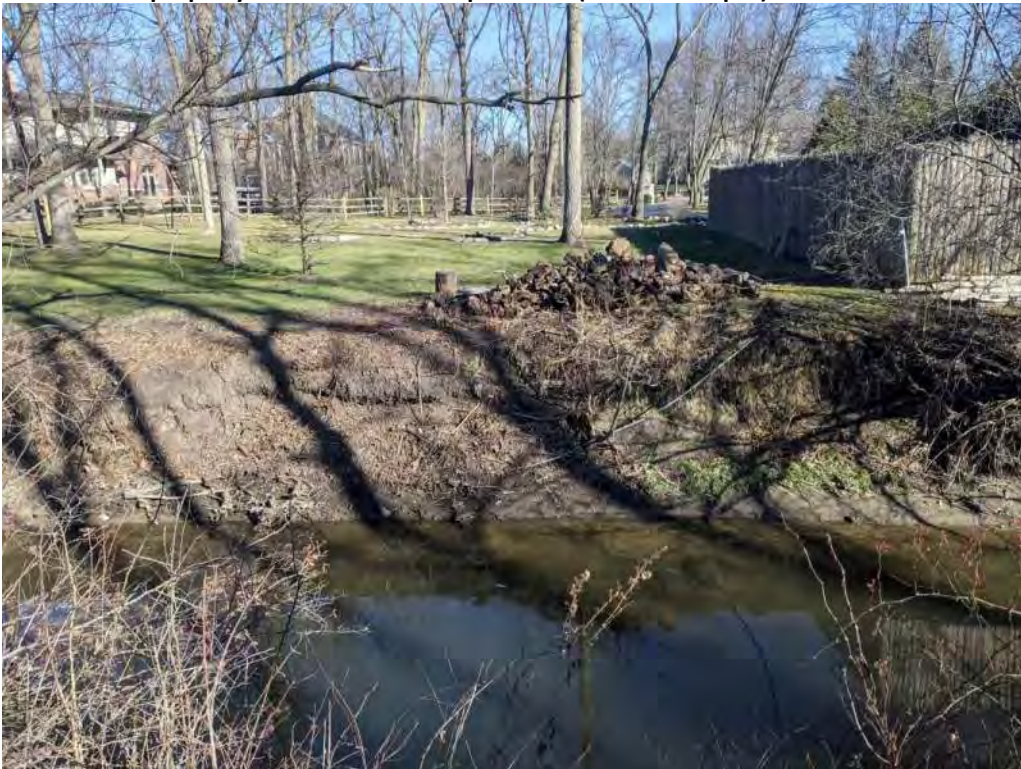
North end of property – 6 to 7 feet of steep erosion (0.5:1 or steeper)
