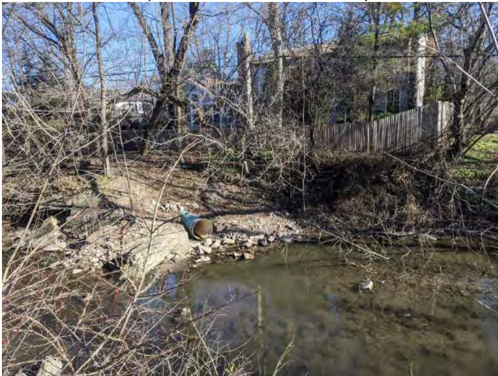
South end of property – 6 to 7 feet of steep erosion (0.5:1 or steeper) with fence at top of slope. - Slope on 211 Glenwood – fence is owned by 710 Waveland
