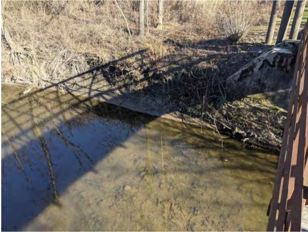
North side of pedestrian bridge from top – 4-5 feet of vertical erosion (0.5:1 or steeper)
