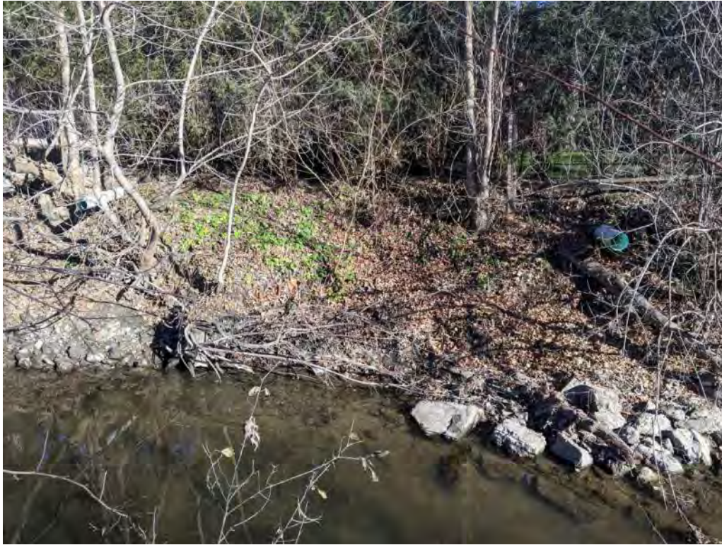
South side of property – bank erosion – driveway at top of slope at risk if erosion continues
