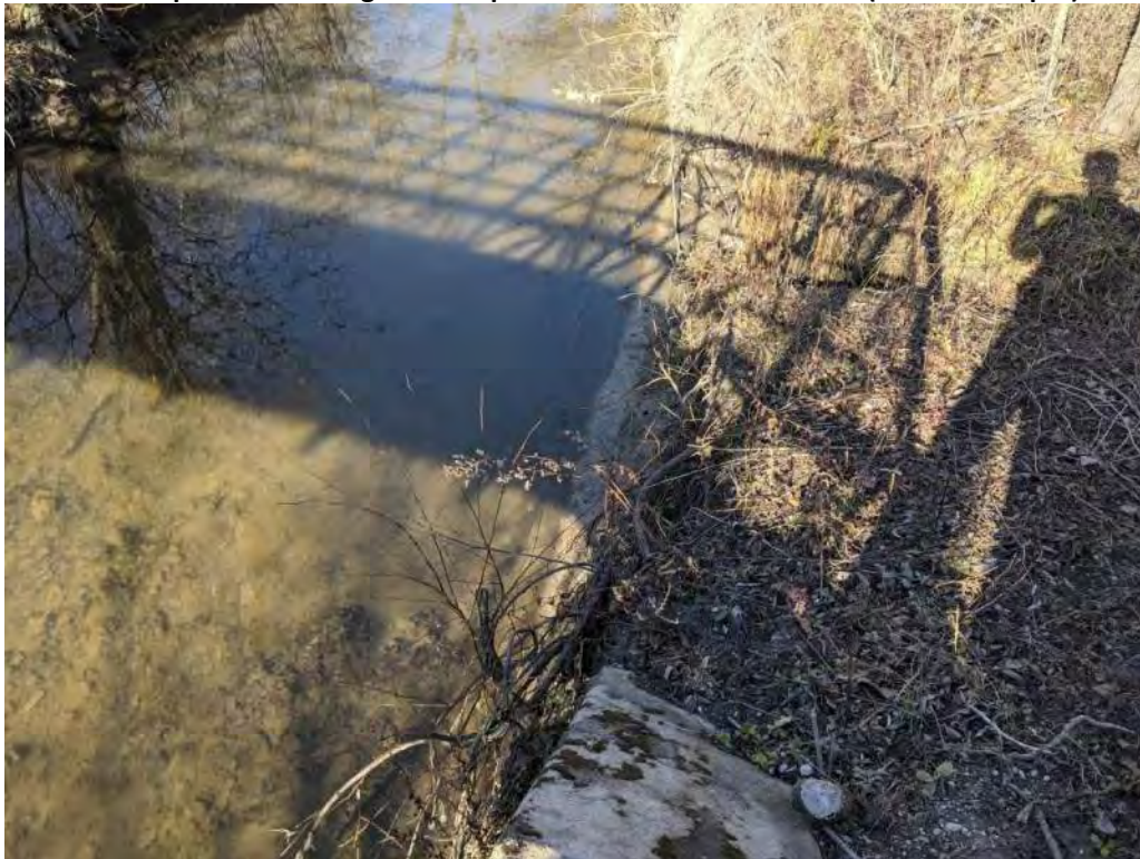
North side of pedestrian bridge from top – 4-5 feet of vertical erosion (0.5:1 or steeper)
