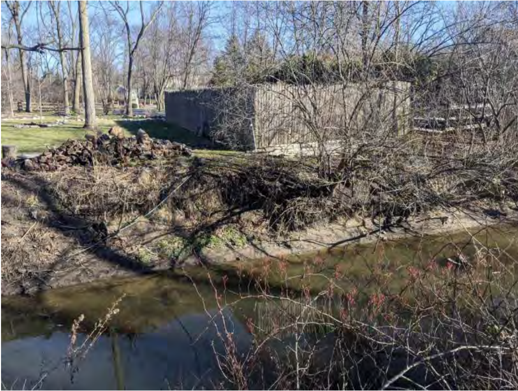
North end of property – 6 to 7 feet of steep erosion (0.5:1 or steeper)
