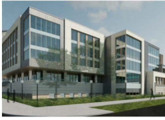
Annex Facade Upgrade Scheme 1
