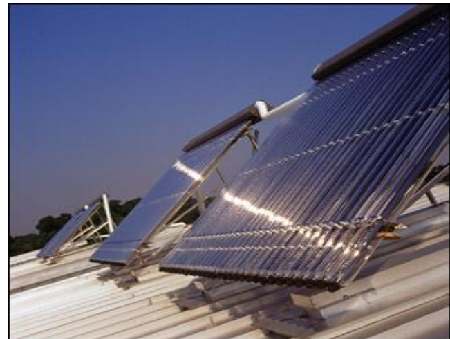
Solar water heating using tubular piping system placed on the roof.
