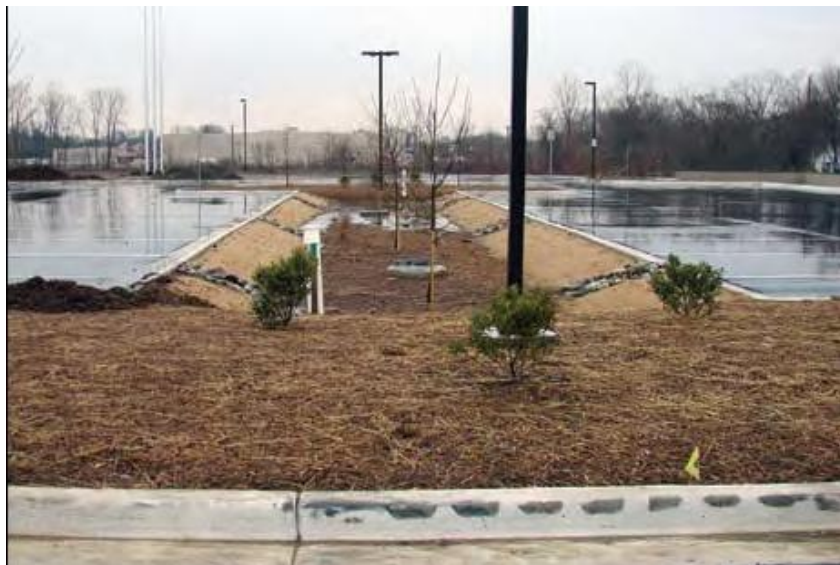
Bio-filter swale under construction.
