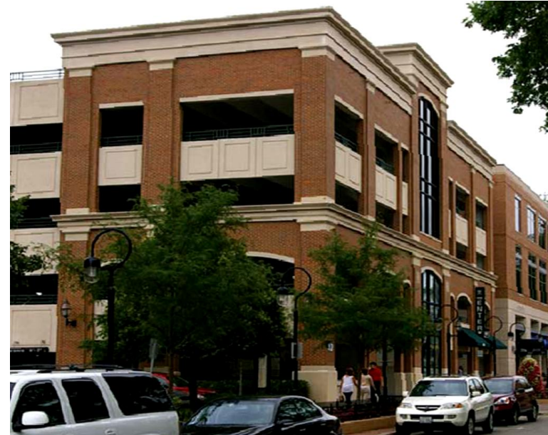
Vertical brick articulation combines with horizontal banding to form grid framework and cornices unify the top of building.
