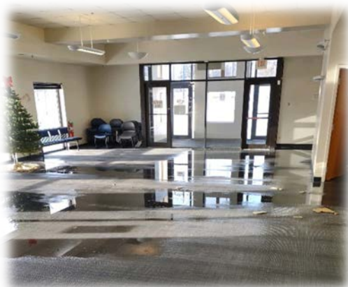
Water Line Break Repairs
