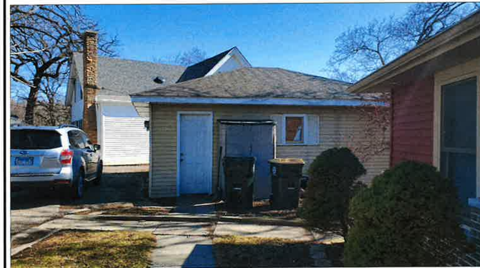
VIEW OF EXISTING GARAGE FROM FRONT WALK OF HOUSE
