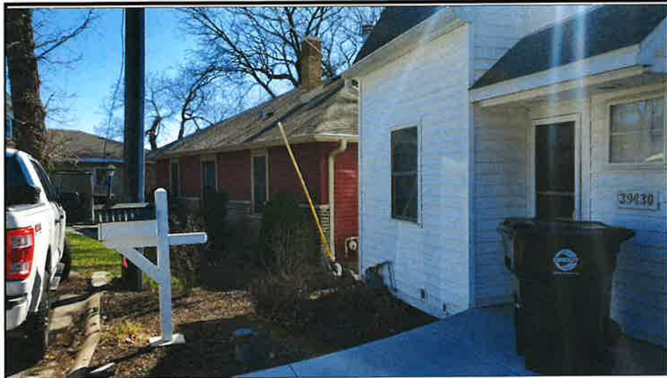
VIEW OF EXISTING HOUSE AND GARAGE FROM NEIGHBOR TO THE WEST
