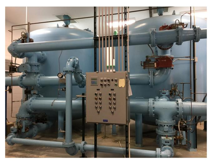
Shown are the two tanks and related control systems in the Lake County Public Works Iron Filter System for the Prairie Pointe water system. A recently awarded contract for \$210,194.00 will replace the layers of specialized sand, gravel and interior piping of the tanks as well as modernize the electrical control systems. Work is scheduled to be completed in June 2018.
