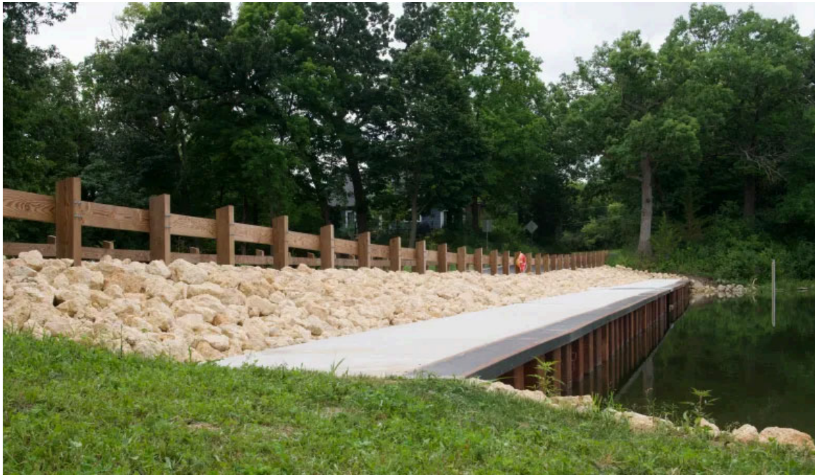
The Sylvan Lake Dam post reconstruction, including a new sheet pile wall. The new dam also now has the ability to dewater the lake, officials said. (Joe States/Pioneer Press)
