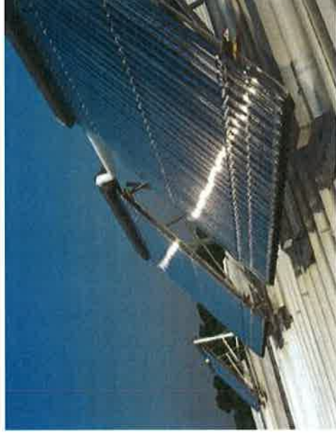
Solar water heating using tubular piping system placed on the roof.
