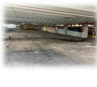
Parking Garage Renovation
