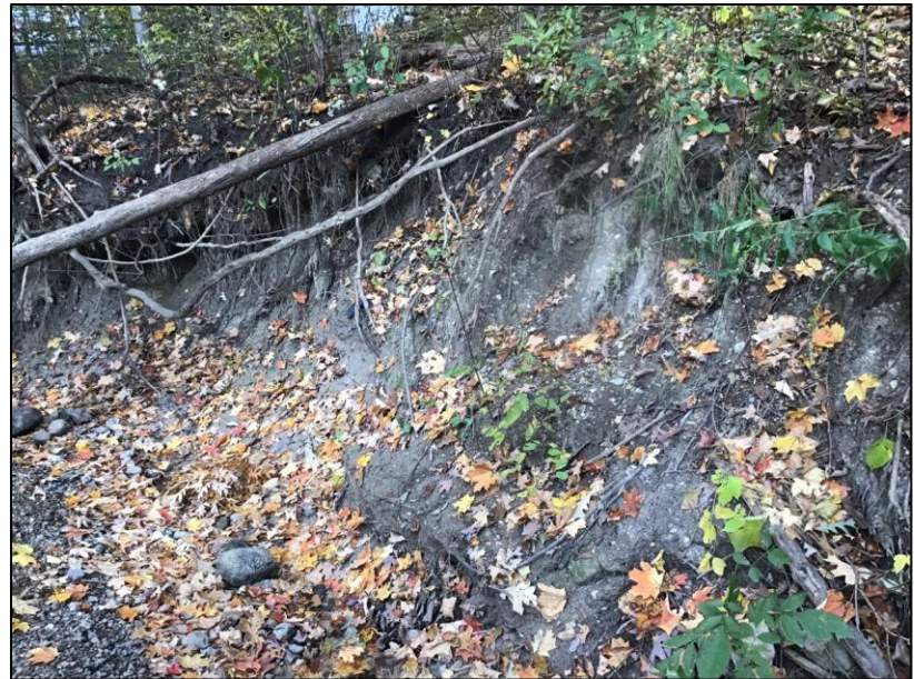
Figure 3-43: Streambank Erosion Example
