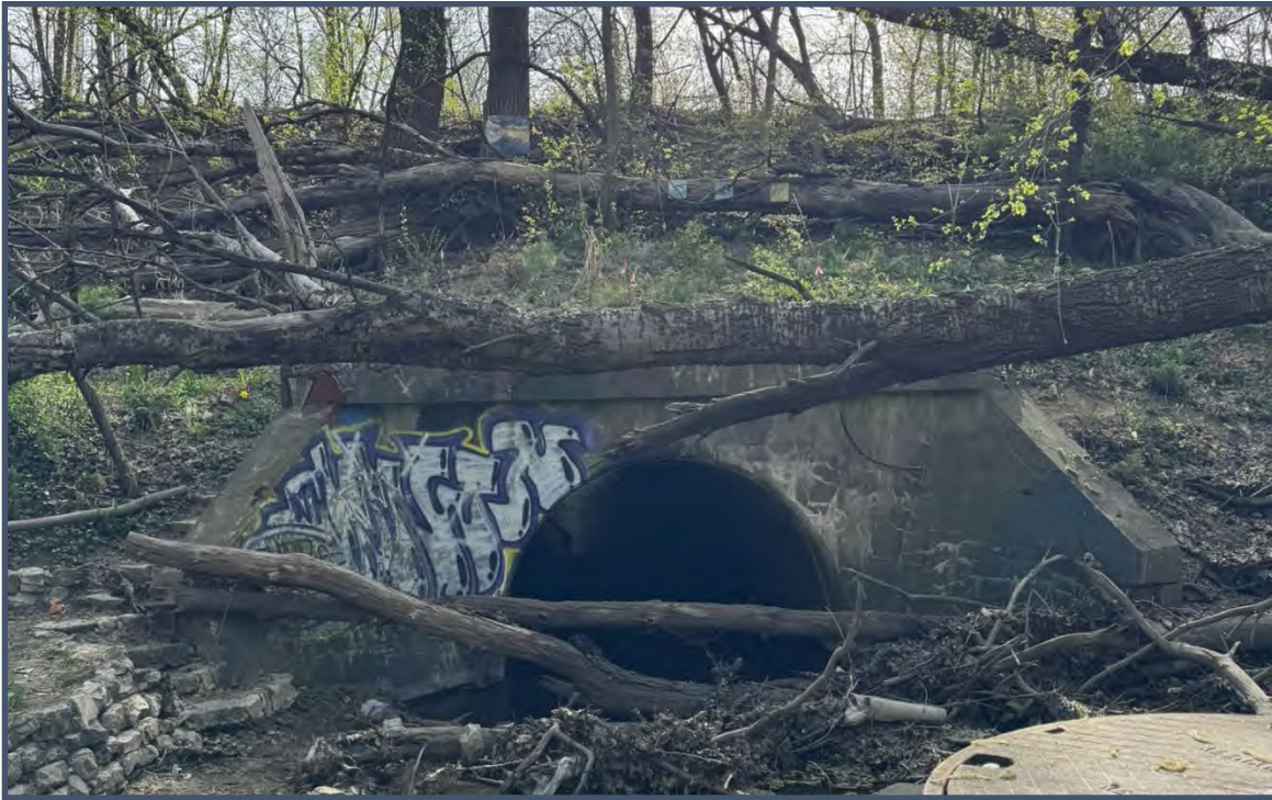
Photograph 1- West Elevation (Looking East at Headwall)
