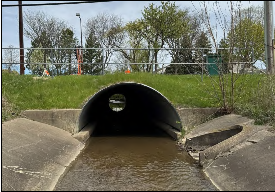
Photograph 1–Downstream End Section (Looking Upstream)
