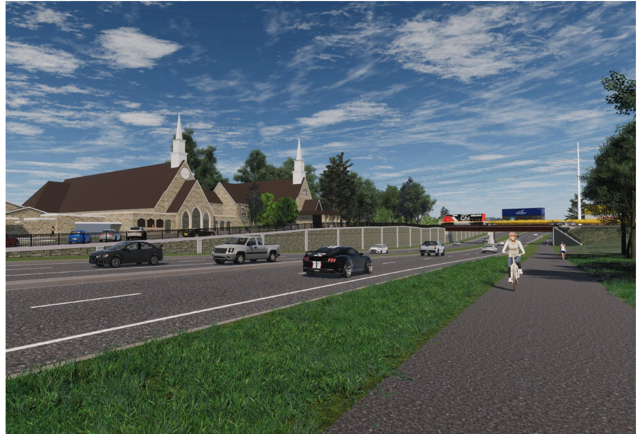
Rendering looking west at new CN railroad bridge over Old McHenry road and St. Matthew Lutheran Church
