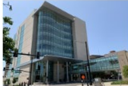
Lake County Criminal Court Tower Waukegan
