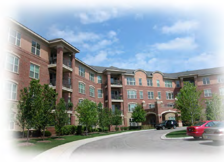
Examples of acceptable Multi-Family facade designs indicating the use of elements such as dormers, wall projections and dominant entry features.
