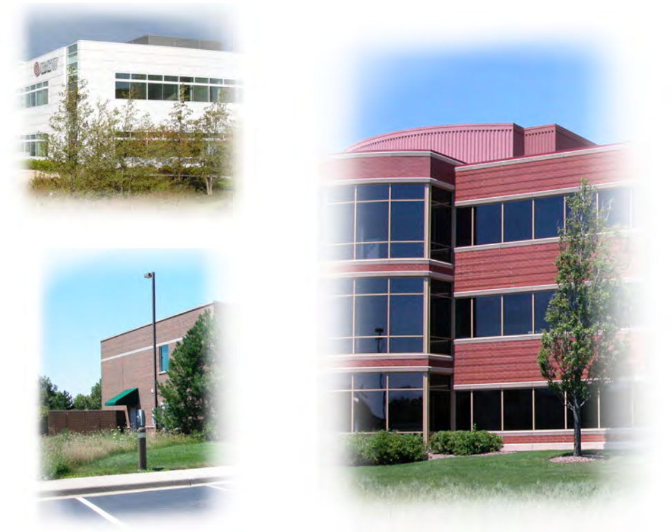
Examples of acceptable screening for mechanical equipment..
