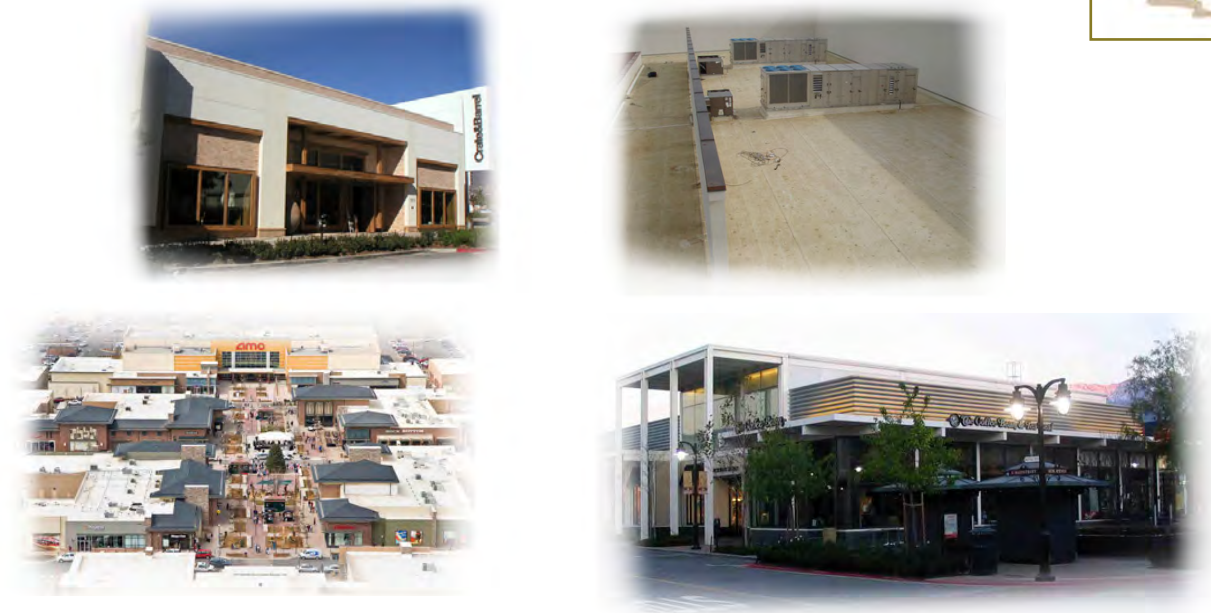
Examples of acceptable screening for mechanical equipment.
