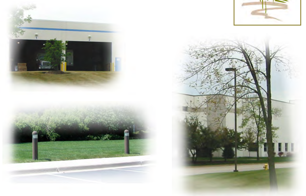
Examples of acceptable building lighting.
