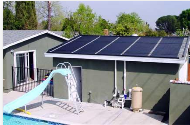
Solar (thermal) pool heating system
