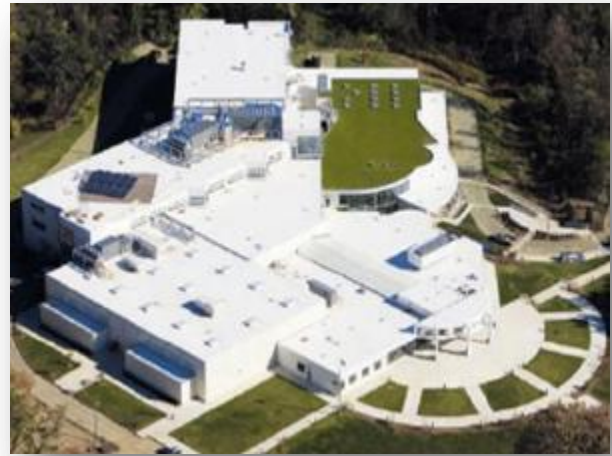
Cool roof and green roof system
