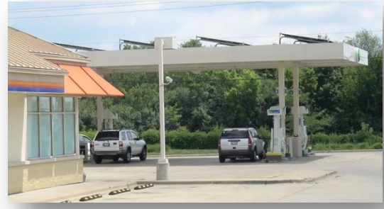
Canopy-mounted solar panels
