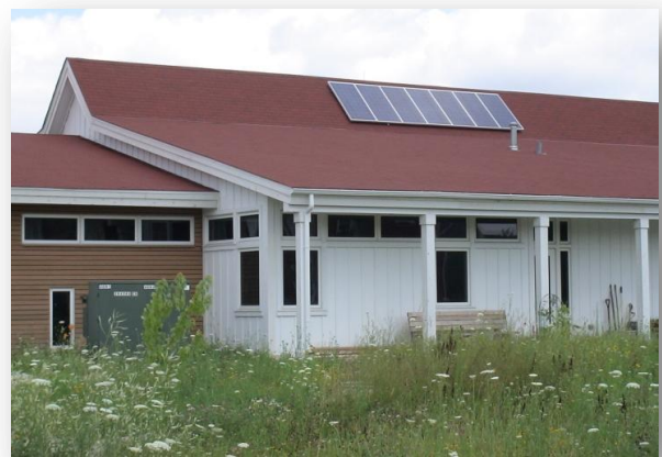
Solar Array on the Prairie Crossing Charter School – USBC-certified LEED Gold.
