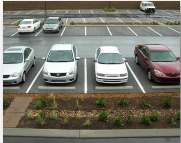
Pervious paving for parking stalls; conventional paving for drive aisles
