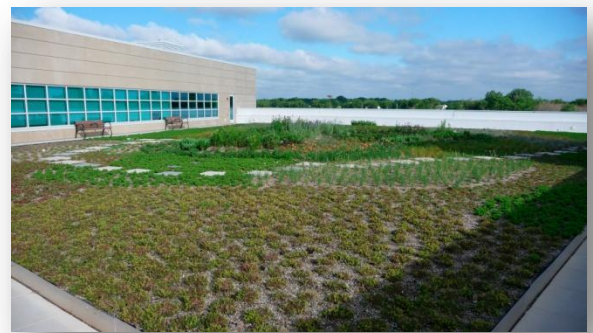
Green roof, Lake County Central Permit Facility
