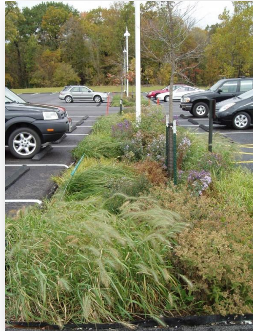
Bioswales in parking lots help filter stormwater runoff. This one is at the Ryerson Woods welcome center – USGBC-certified LEED Platinum.
