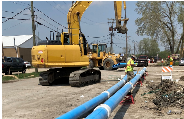
Baker Road Water Main Replacement
