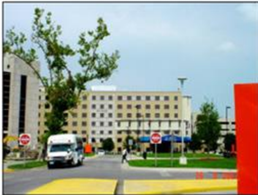
H Bldg East Pavilion (2)
