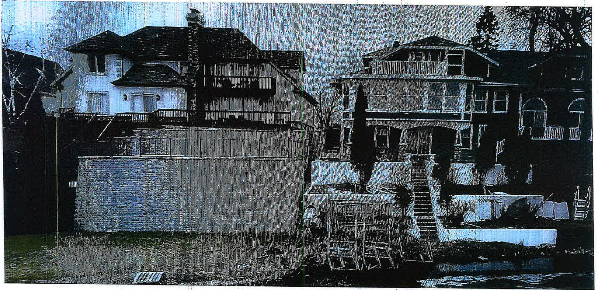
Subject property and neighbor to west showing proximity to water
