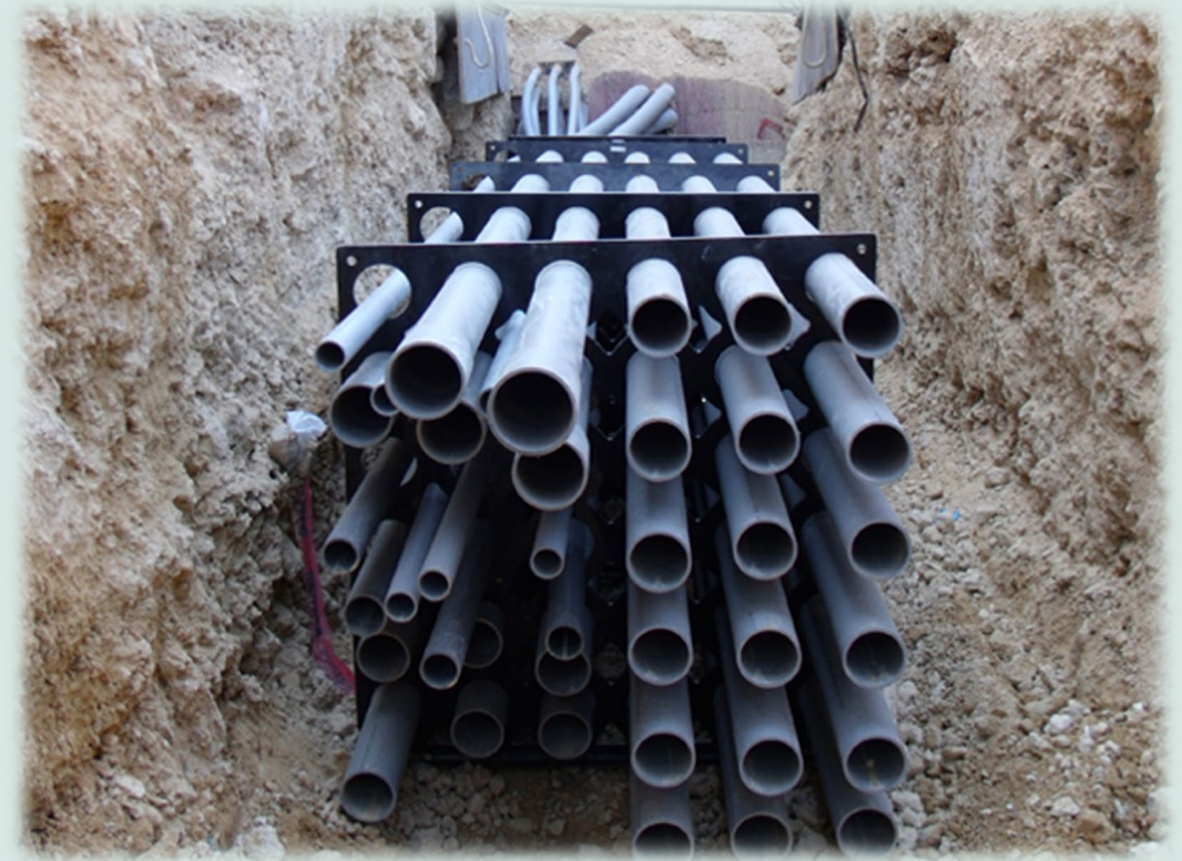
Example of conduit ducts
