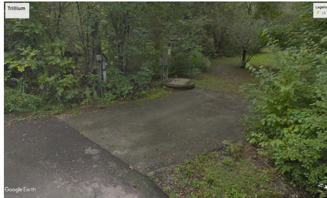
Figure 1- Typical Site Pre-Improvements
