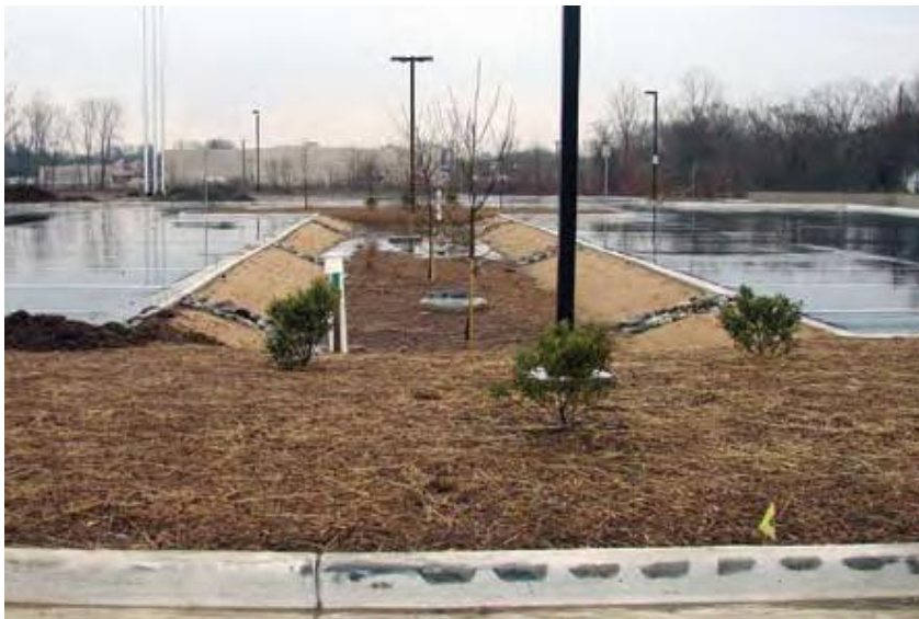
Bioswale under construction.
