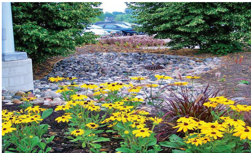
Stormwater basin catches excess flow in parking lot island.
