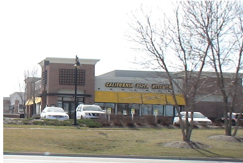
Roof elements hide mechanical equipment.
