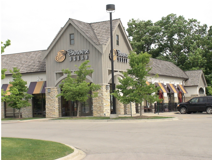
Encouraged: Use of roof structure to hide mechanical equipment.
