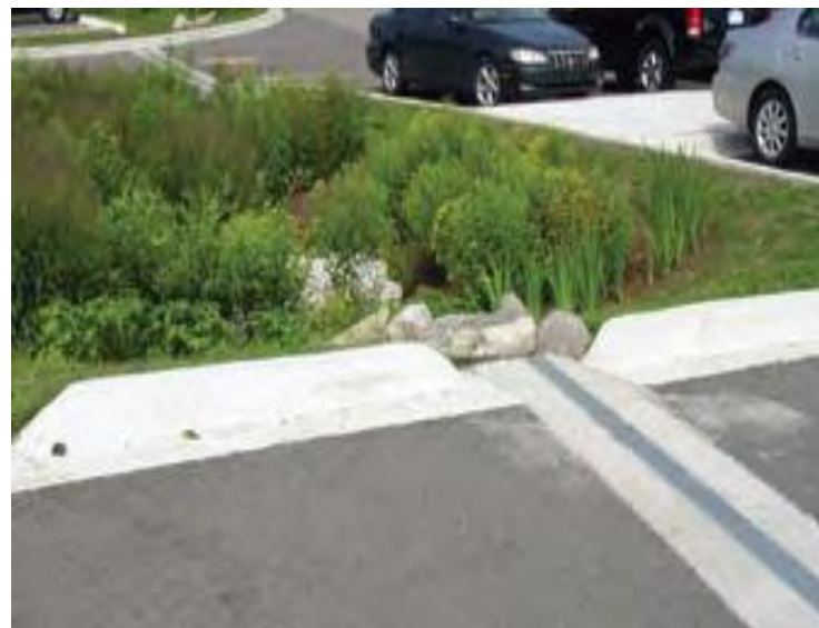
Interior parking island with overland flow into swale.
