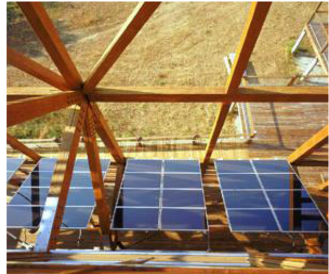
Solar panels incorporated into building elevation/roof top.
