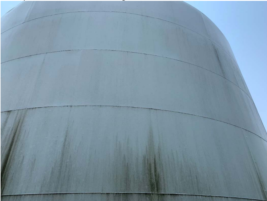
Bradley Road Water Tower Washing
