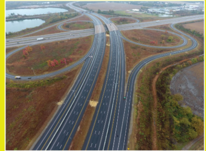
Interstate 255 reconstruction between I-55/70 and Illinois 15, St. Clair County, IL
