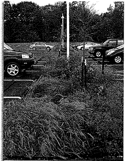
BIOSWALES USED IN PARKING LOTS, LIKE THIS ONE AT THE RYERSON WOODS WELCOME CENTER, A LEED PLATINUM FACILITY, FILTER STORMWATER RUN-OFF AND POLLUTANTS.
